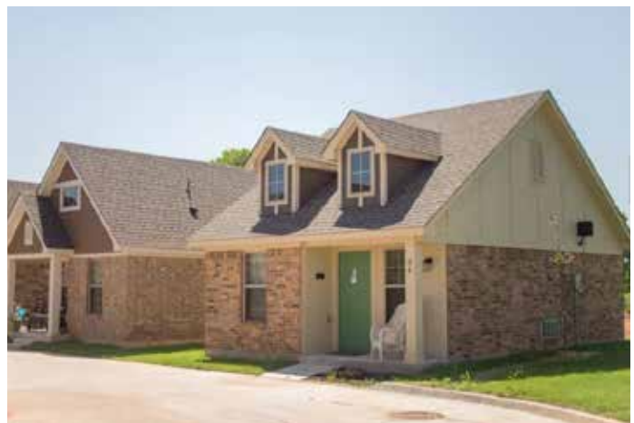
Tiny houses for individuals (top) and families at Food and Shelter in Norman, Oklahoma
